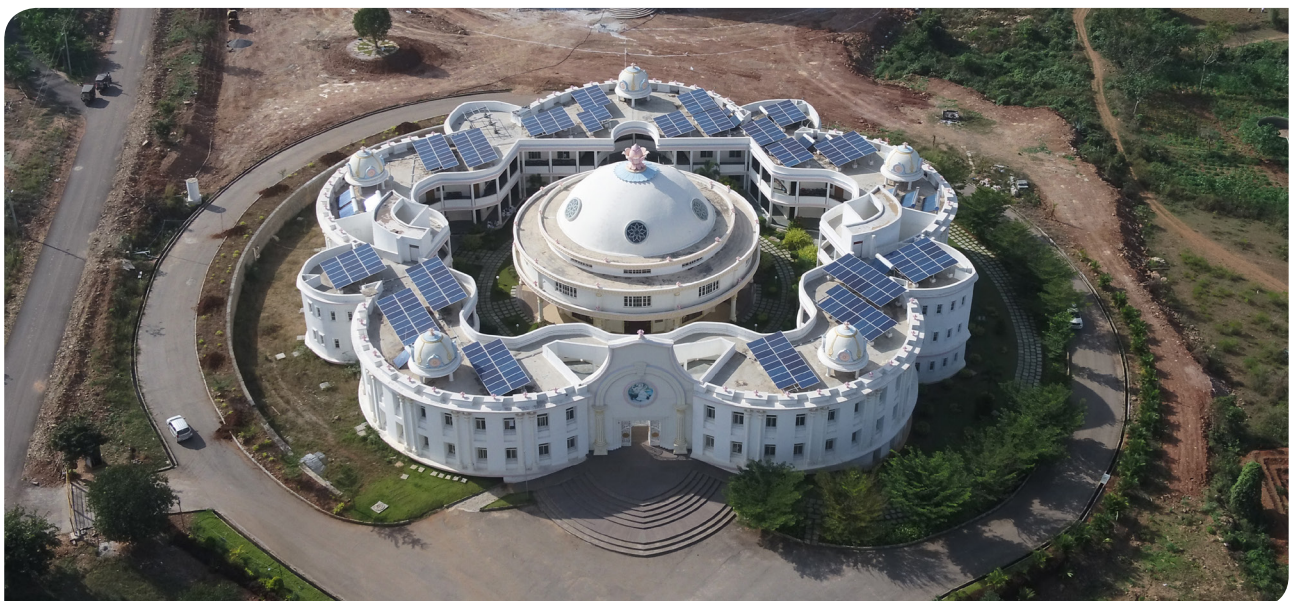
Solar Panels established in our campuses for efficient use of energy
